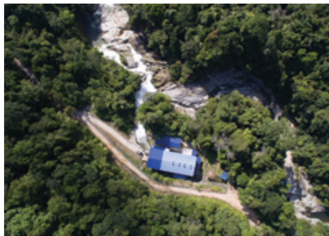
Amcorp Perting Hydro 6MW, Bentong, Pahang.
